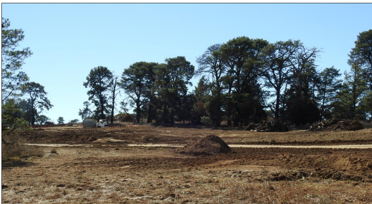
Plate 2-1: Monterey pine stands and vegetation clearing for pipeline construction, August 2017
